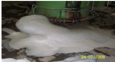
Severe foaming at CW Pump and in CW Foreway due to organic contamination
