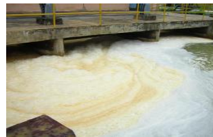
Severe foaming at CW Pump and in CW Foreway due to organic contamination
