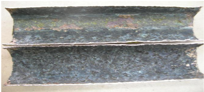
BIOFOULING OF Cu/Ni CONDENSER TUBES
