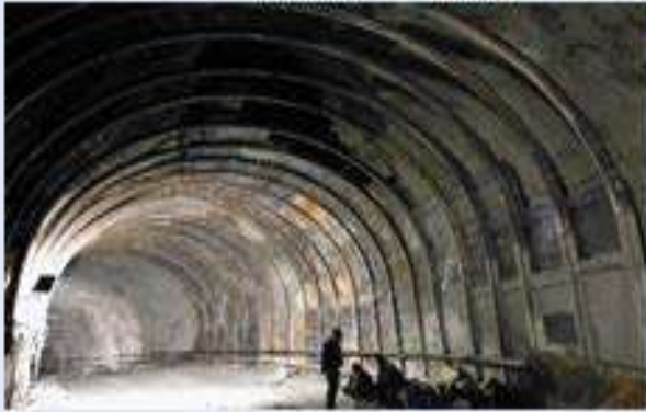
Main Access Tunnel of 1000 MW Pakal Dul HE Project
