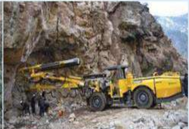
Drilling Machinery/Equipment at Pakal Dul HE
